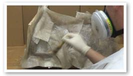
As before I take care of the tricky areas first with a layer then hit the whole surface with two layers of glass and tap them all down, one layer at a time.
